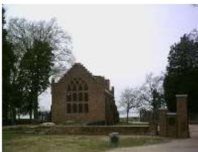
Exterior of the 1907 church (with graveyard in left foreground)
